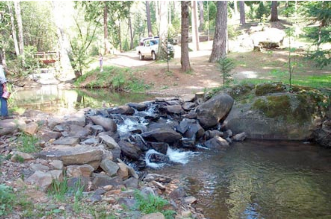
Another aeration structure between two pools.
