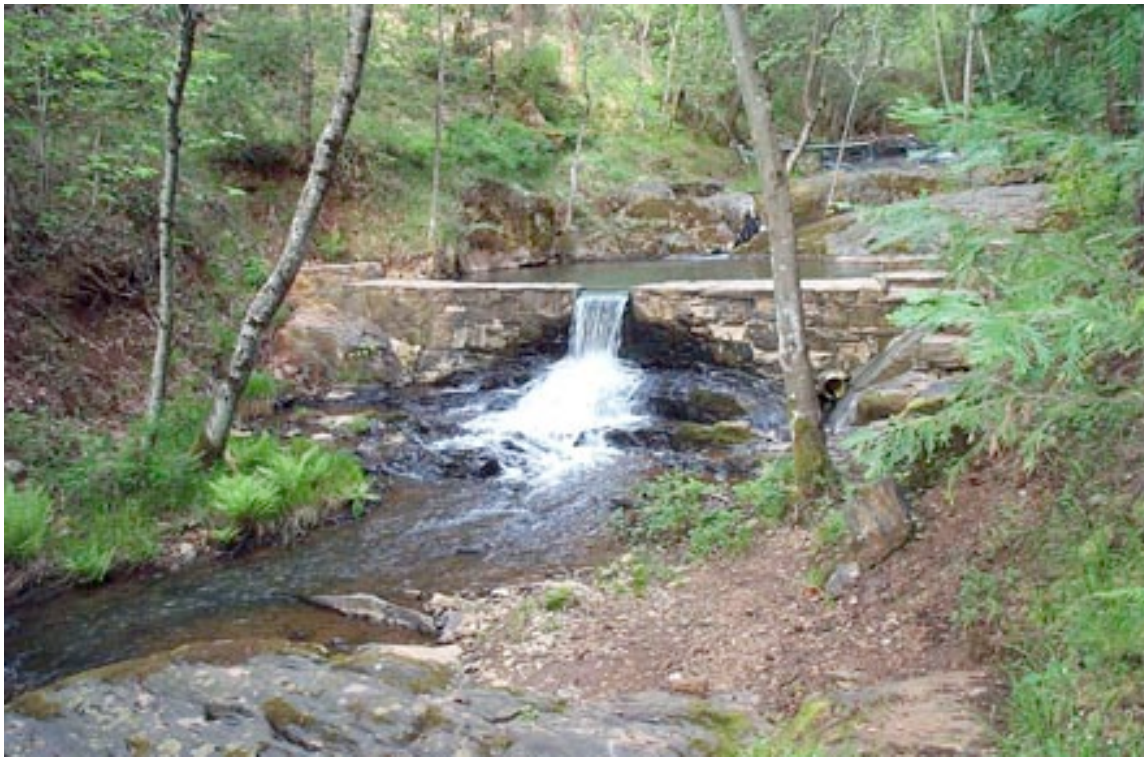
The small dam creates the pool upstream.
